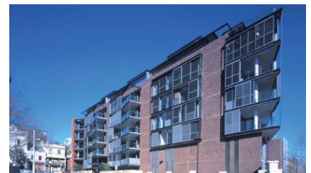
Figure 22: Walsh Bay Apartments (Mirvac) Example building design showing setback upper storeys, defined street wall and articulated façade.
