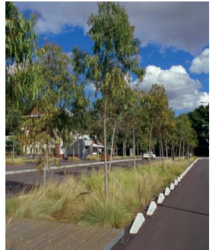
Figure 25: Example of water sensitive urban design in the public domain (top) and within the street reservation (below).
